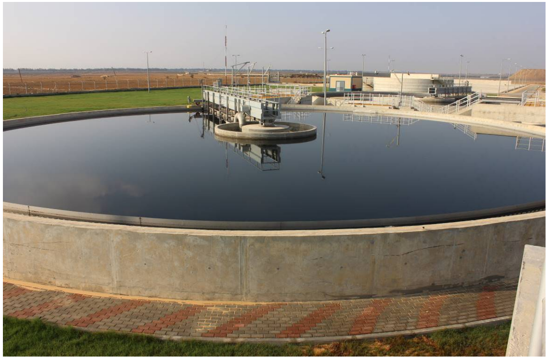
Clarifiers Filled with Purified Waste Water up to December 2019
