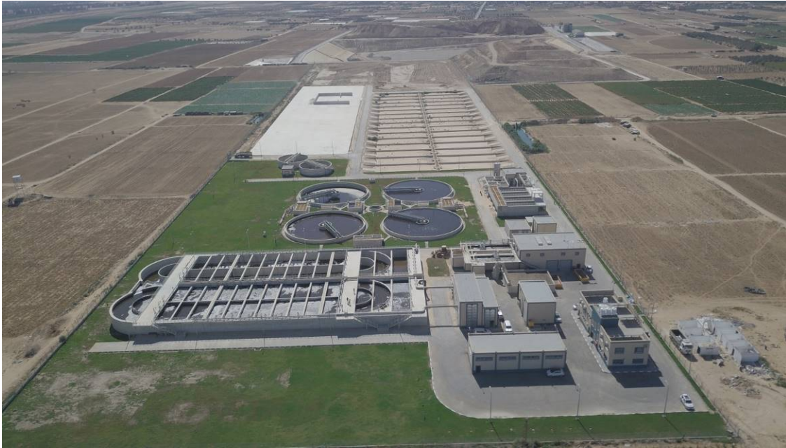
General Overview for KY WWTP Filled with Waste Water in December 2019
