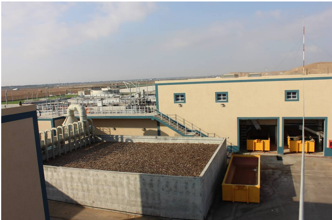
Bio-filter for Treatment of Odour from the Pre-Treatment Building up to December 2019
