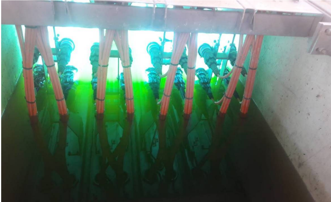
Ultra Violet Disinfection of Treated Effluent in the Sand Filter up to December 2019
