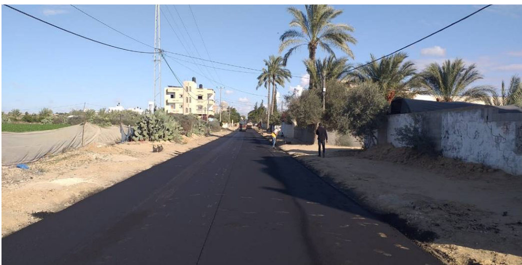
Asphalt Work in Road No.14 in Al Fukhari up to December 2019
